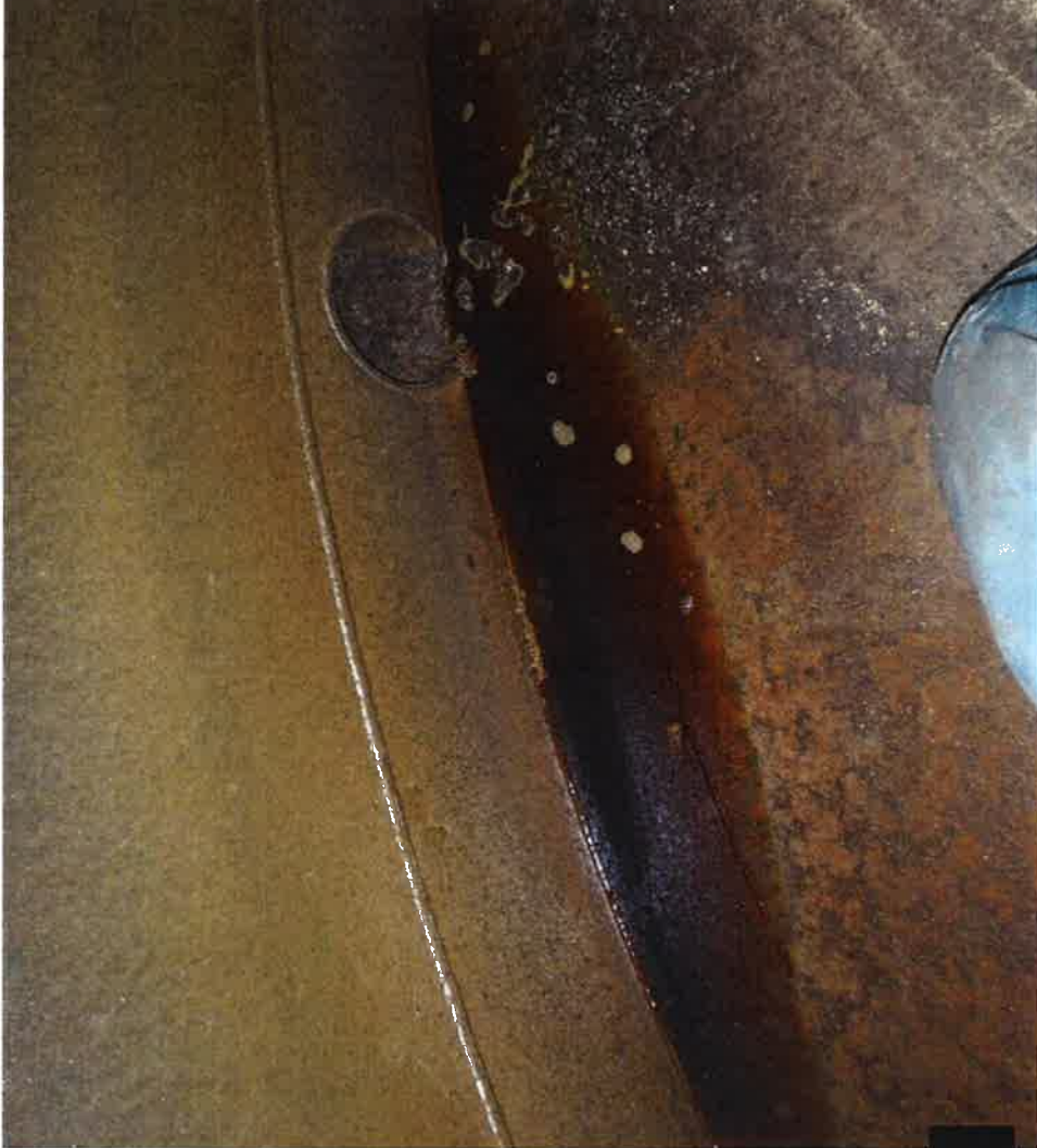
DRAIN PLUGGED IN STACK ON SUB FLOOR
